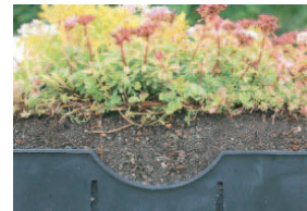
B Green Roof
