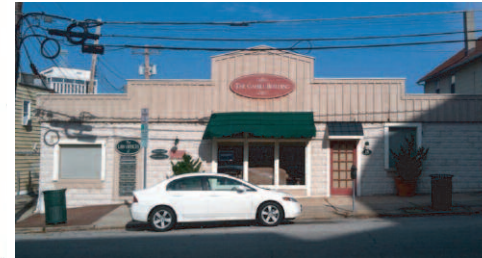
Existing Conditions – 15 E. Chesapeake Ave.
